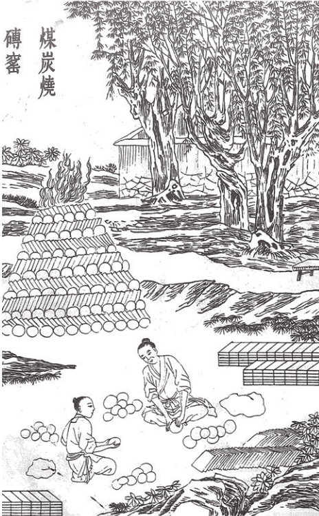
Fig. 8. Drawings from Tiangong kaiwu [Creations of Nature and Man] of Chinese tile and brick production sequences in the seventeenth century: (top left) producing brick by mud; (top right) making tiles by barrel-molding technique; (bottom left) using coal to fire bricks in the kiln; (bottom right) pouring water on the top of the kiln to create an oxygen-deficient environment (from Song 1998:225–228).
